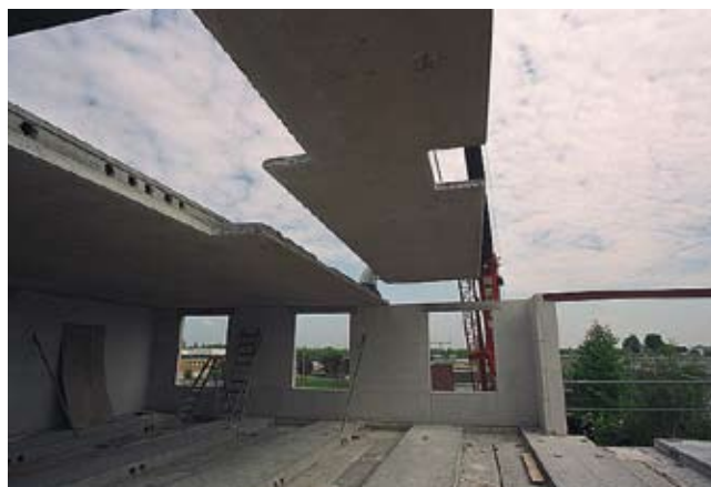
Montage Wing-element.
